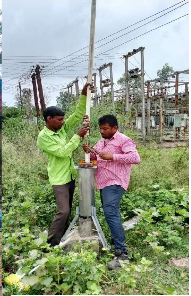
Installation of hand pump set at Project affected Villages
