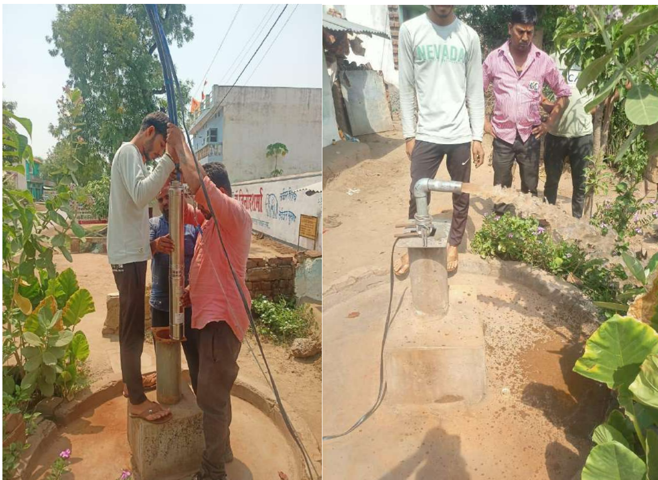
Installation of 5 HP Submersible pump at Project affected Villages
